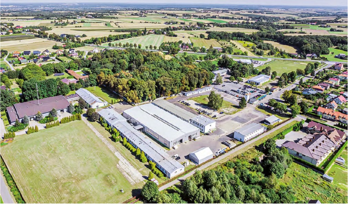
Luxiona Main Factory, Jacentow. Poland
