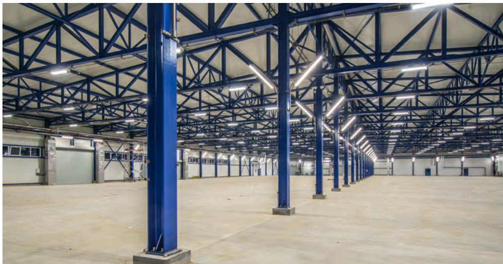
Nitrogen Plant, Pulawy, Poland
